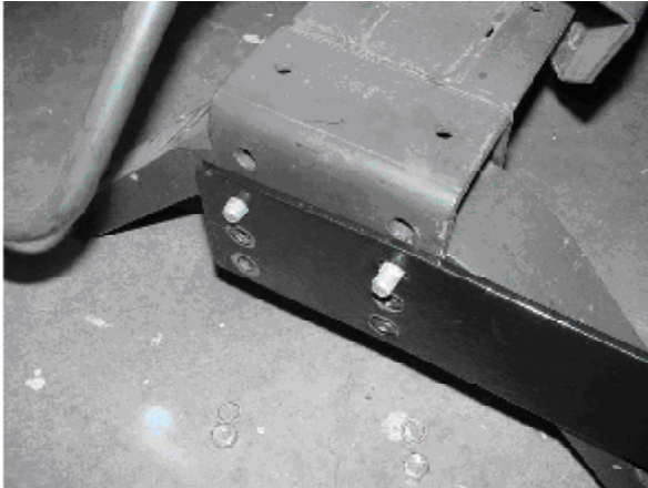
Figure 3-Left Side Plate installation
