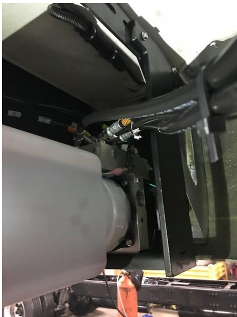
Pump mounted on bracket
