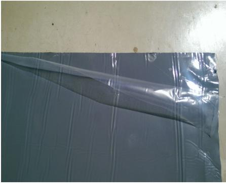
Peel back 1" of clear liner 8" in length. ( be careful not to let the gray adhesive material come in contact with its self ) it will be very hard to get apart.
