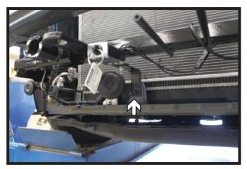
13. **Optional Breakaway:** Using a 12MM socket, remove the existing screw and reinstall with the breakaway bracket. Install the breakaway switch to the bracket with the supplied 1/4" hardware.
