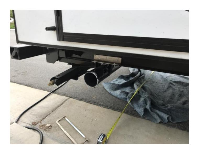
Here is the passenger side pipe after its mounted and cut. I needed 94" from the box to the end. This 94" was total and included the ABS cleanout I installed which is on the next page.
