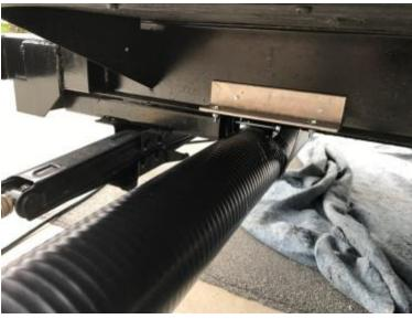
Here is the mock up. In this middle picture I just have the pipe fitting on the back of the box supported on the bracket. Its hard to see the vent pipe hangars because I painted them black. Next page has a blown up picture and you can see the vent pipe better. In the bottom picture you can see the brackets better. I ended up cutting the pipe after I installed the passenger side to ensure I got it fit perfectly.
