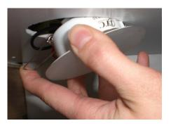
4. Installing the screw mount version: Remove cover by twisting counter clockwise. Mark location of screw holes and pre-drill. Using screws provided, screw in fixture and re-install cover by twisting clockwise.
