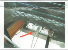
6. Connect the 3-pin connector to the control box, if installed.
