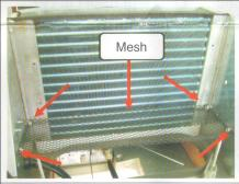
4. Install mesh screen (reinstall screws from step 3 and add (2) additional screws in locations shown).
