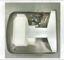
1. With the AC on a flat surface, remove outer shroud.
