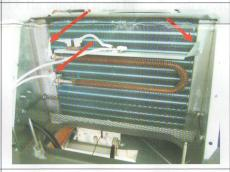
5. Install heating element using provided screws.
