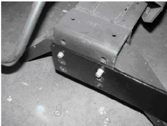
Figure 3-Left Side Plate installation
