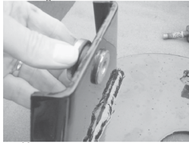
Figure 20 – Installing Thick Bushing
