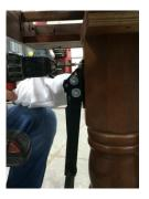
8. Carefully pull Chair Buddy<sup>TM</sup> T-Handle down. Using the provided screws secure the top mounting holes.
