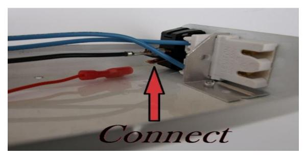
4. Connect the LED tube cord into 1 of the 2 snap connectors (either one). (The extra snap connector is for fixtures that use two tubes.)
